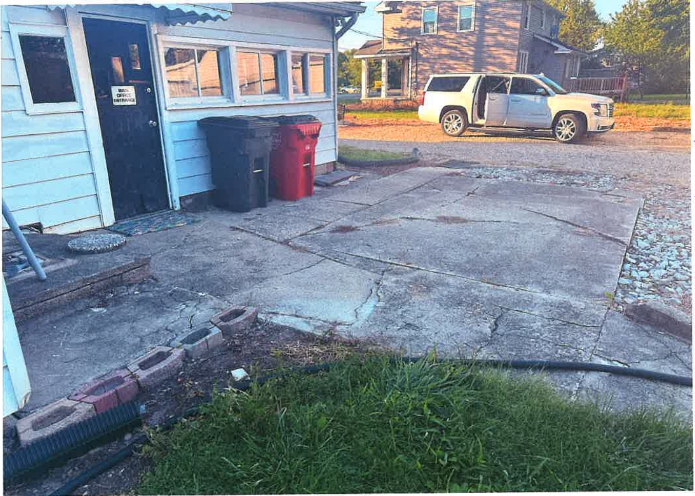
New concrete ordered
